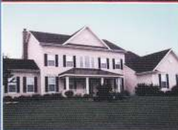
The Summit – Hawthorne Woods, Illinois Install James Hardie 8 1/4" cedarmill cement lap siding with two coats of acrylic stain.
