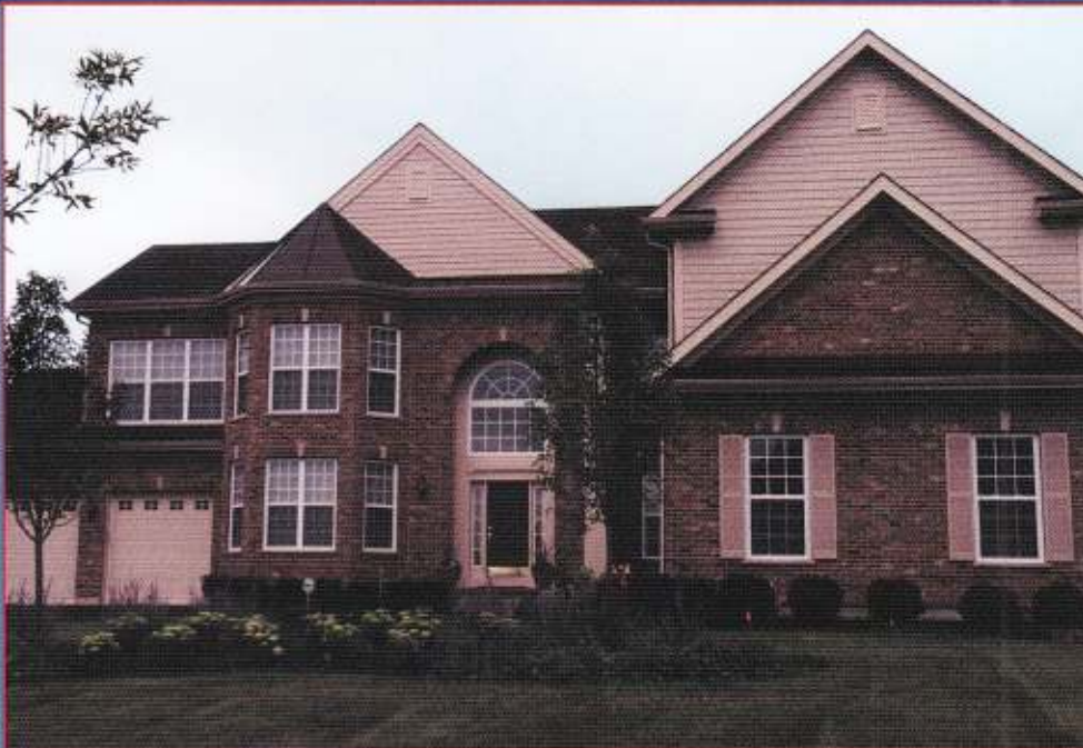
The Summit – Hawthorne Woods, Illinois Install James Hardie 8 1/4" cedarmill cement lap siding with two coats of acrylic stain.
