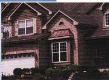
Install Reynolds .019 pre finished aluminum siding and pre finished aluminum soffit, fascia and gutter.
